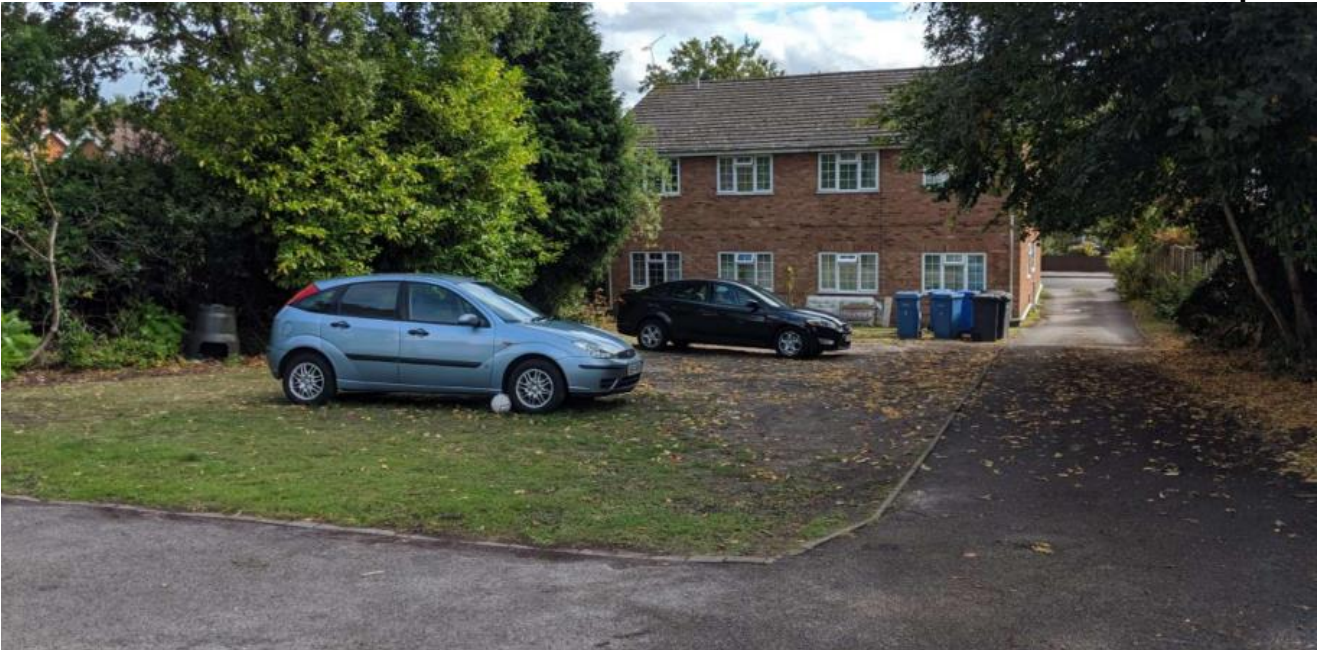
Figure 144 - Existing Rear Elevation of 84 Connaught Road.
